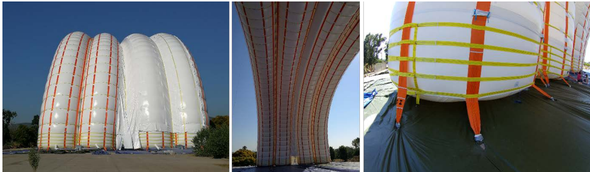
Figure 1. Membrane-strap-anchorage system
