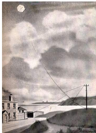
Figure 2: A drawing of the kite aerial used at Signal Hill for reception of the first transatlantic wireless signal. [3]
