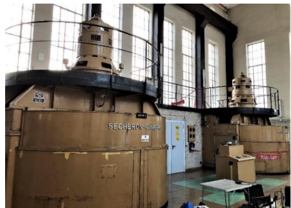
Fig. 1. View of the hydropower plant
