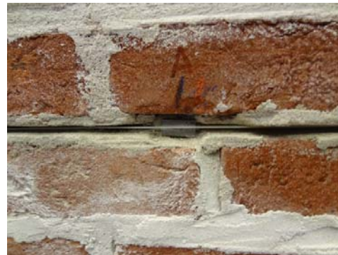
Figure 2: Anchor point and optical fibre in the mortar joint before repointing
