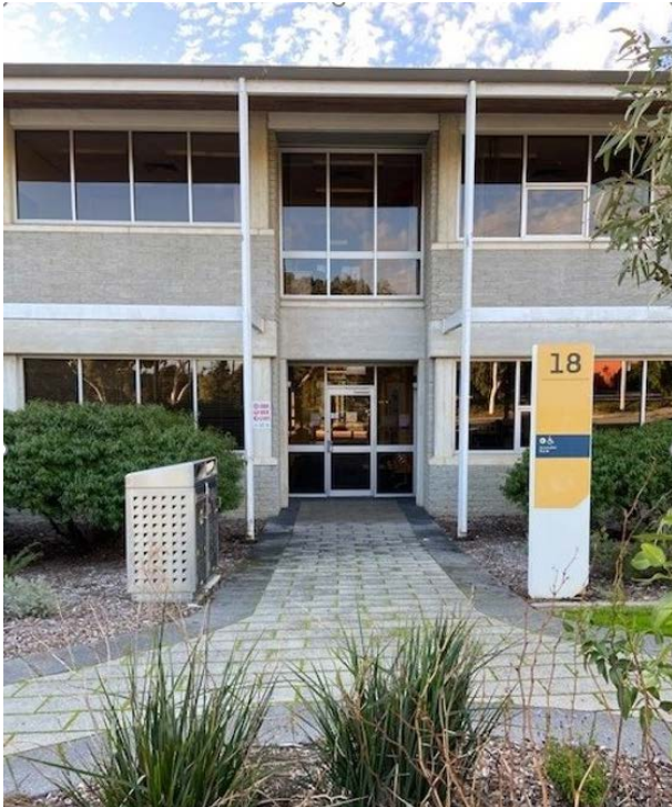
Figure 10: Building 18 exterior view, ECU.
