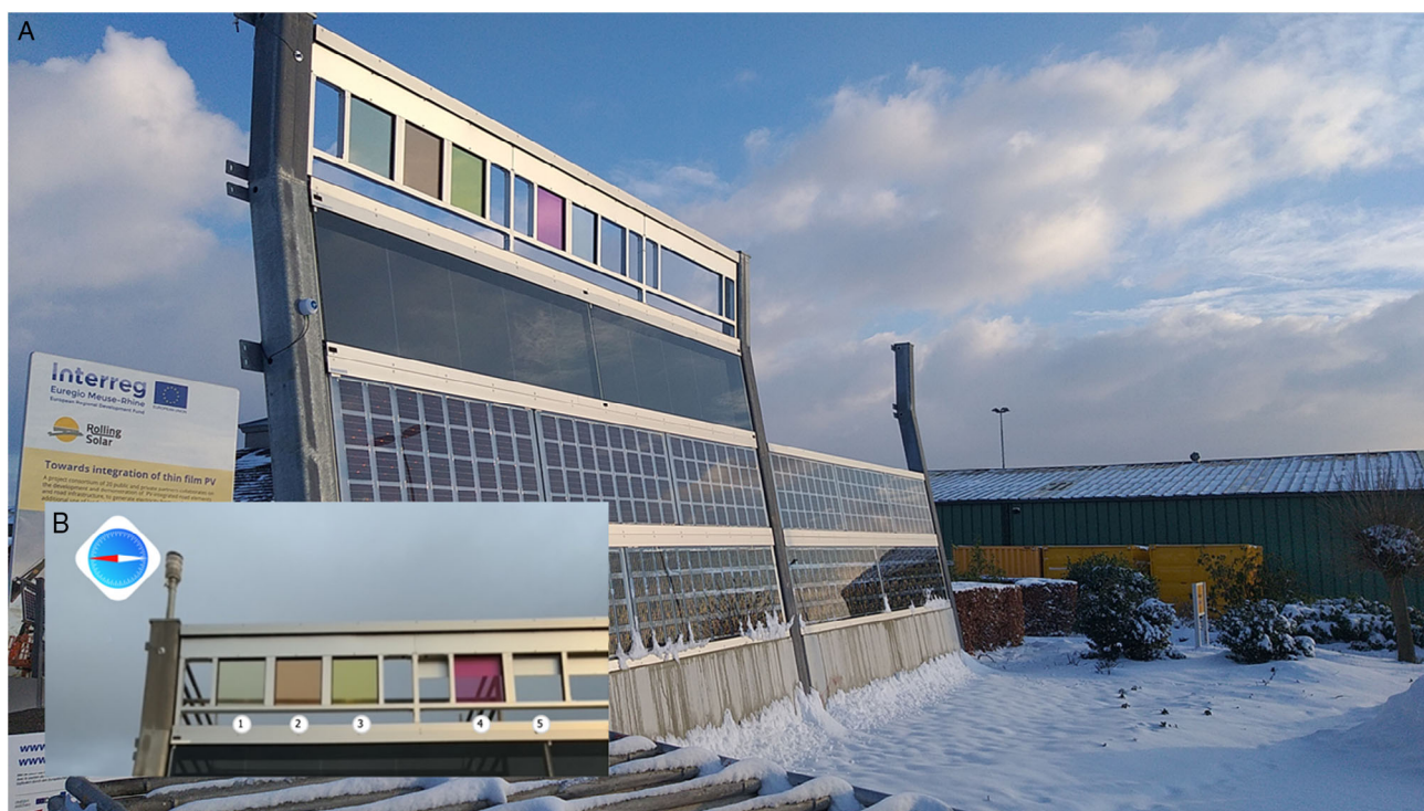
Figure 2. A) Test setup near Rosmalen in The Netherlands, the tinted rectangles at the top of the structure are the LSCs described in this article. The photo was taken on 10 February 2021. B) The orientation of the LSC support structure, the numbers correspond to the following luminophores: 1) InP, 2) CuInS 2 , 3) CdSe, 4) Lumogen, 5) Blank. The red arrow of the compass at the top left of the picture points toward the geographical North.
