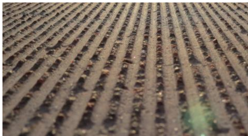
(a) Concrete Otto Alte Teigeler (OAT) Grinding. (Otto Alte Teigeler ,2017)
