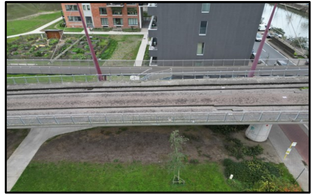
Figure 6: Gaardeniersbrug, Ghent, Belgium. Typical UAS Image of the initial photogrammetric flight.
