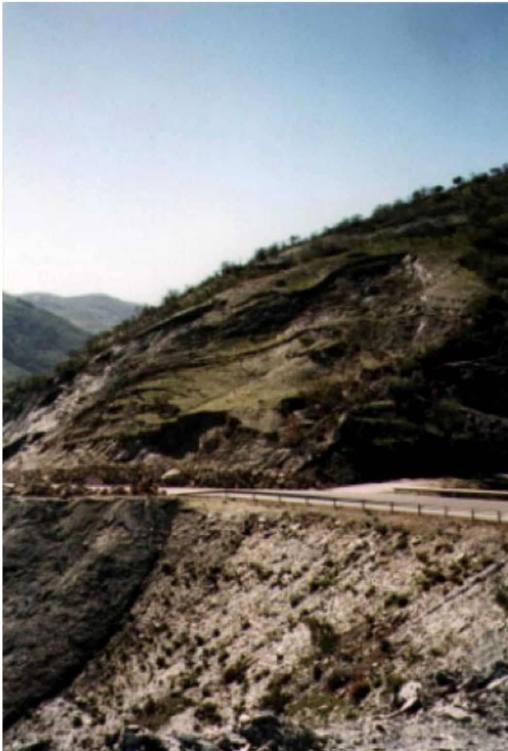
Fig. 1. Torvizcón landslide after the event of February, 1996.
