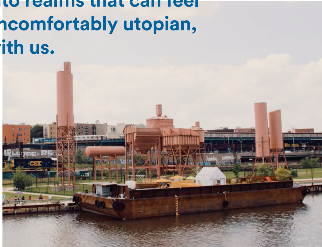
Swale docked at Concrete Plant Park in the Bronx, New York. Photo courtesy of RAVA Films.
