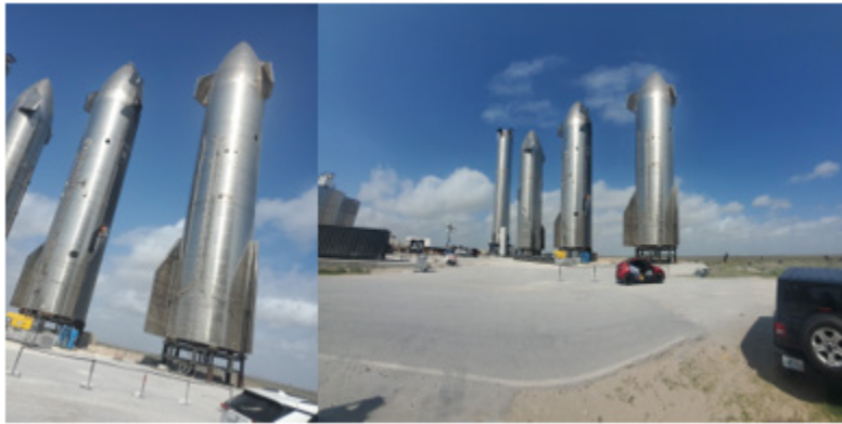
Figure 2. SpaceX Launch Facility Brownsville, TX 80
