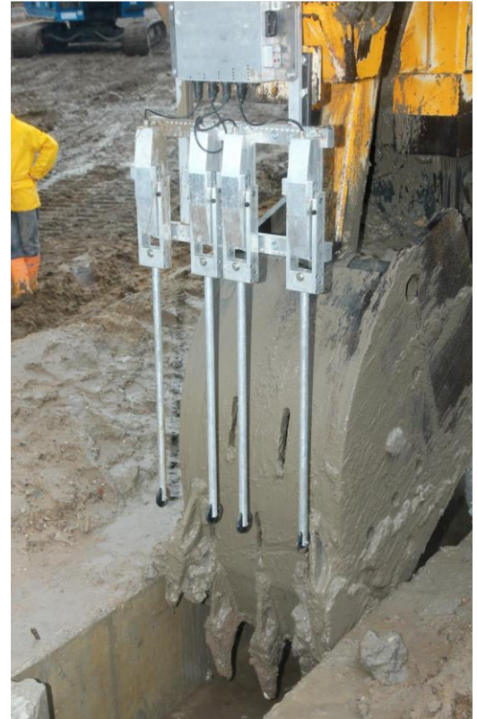
Figure 2.8: Quality control the joints with the joint inspector method
