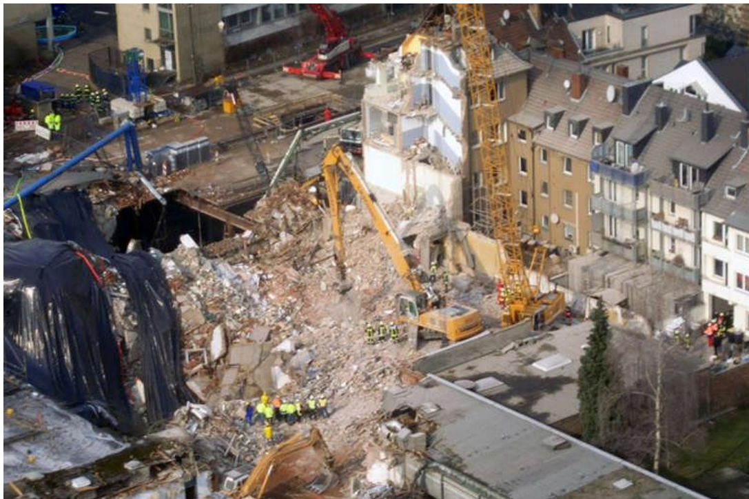
Figure 1.2: Collapse of the Cologne's historical archives ( www.stadt-koeln.de , 2009), ©Stadt Köln/Jürgen Schütze
