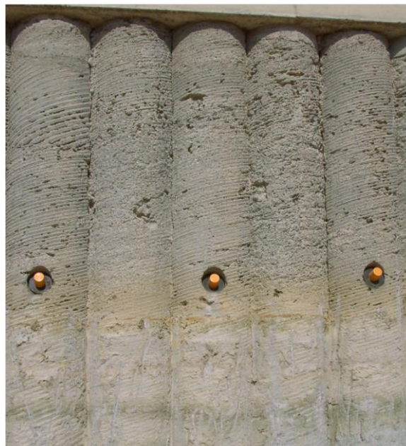
Figure 2.17: Acceptable Imperfections (reprint from (EFFC/DFI Guide, 2018))
