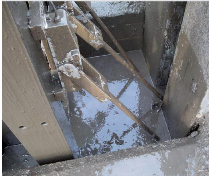
Figure 2.8: Quality control the joints with the joint inspector method
