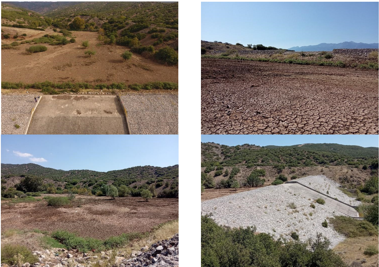
Figure 2. View of the Platana sediment retention dam features: perspective view of downstream slope (face) ( upper left panel ), upstream slope ( upper right panel ), reservoir ( lower left panel ), perspective view of the spillway and crest ( lower right panel ).
