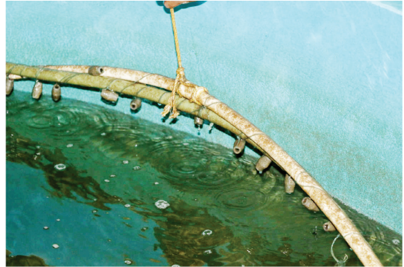
Figure 9. Cleaning of aeration pipe line
