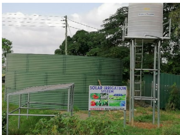
Figure 4: Solar irrigation system at Kwadaso
