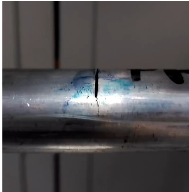
Figure 17. Detail of the notch and the crack of one of the shafts.
