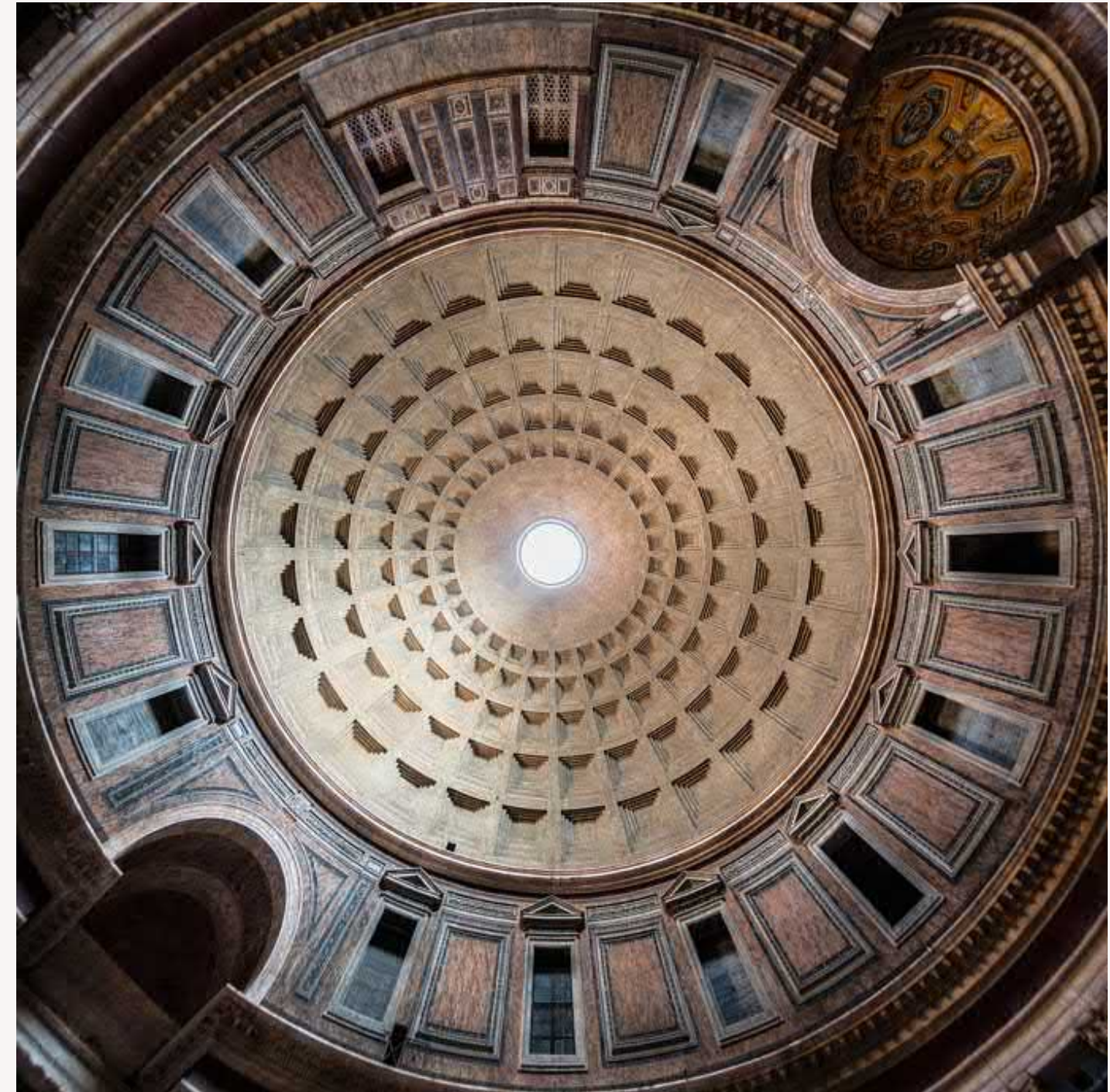
Inside vision of concrete dome structured by intersecting arches, circa 100 AD, Pantheon, Rome. Source: Mohammad Reza Domiri Ganji - Own work, CC BY-SA 4.0, < https://creativecommons.org/licenses/by-sa/4.0/deed.en >, via Wikimedia Commons.
