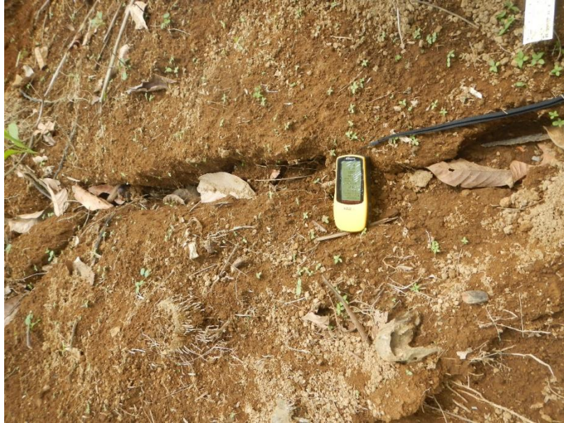
Figure 3.6 Small trench or rill formed due to intensive soil erosion process in Bompon watershed.
