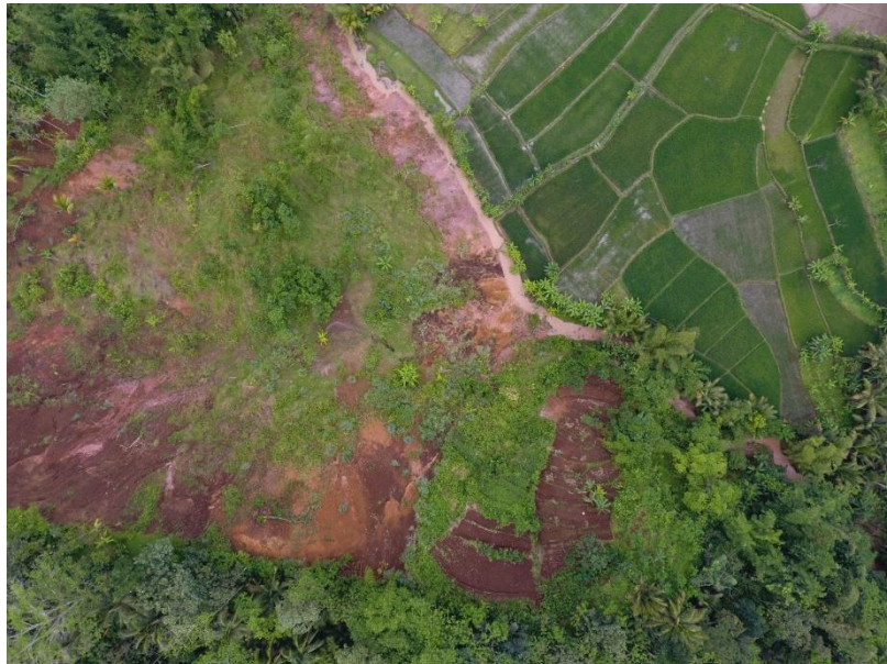
Figure 3.7 Aerial photograph of the largest landslide site in Bompon, located in Kalisari Village. The landslide process starts more than 10 years ago and still expanding, threatening the paddy field and road infrastructures.
