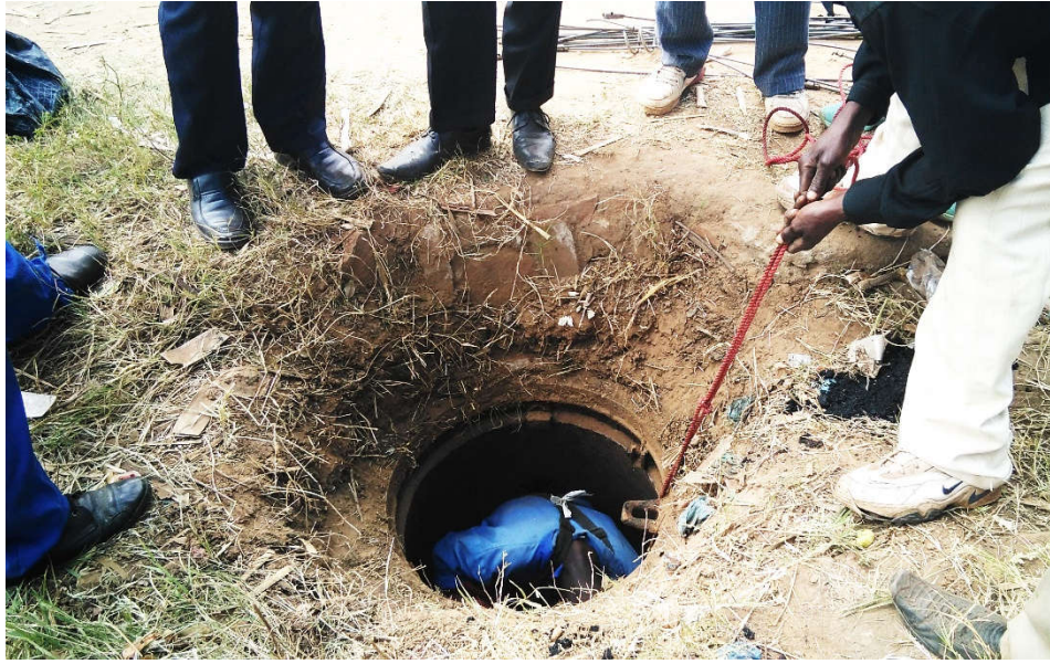
Figure 17 Sewer worker going into a manhole. Image: Author's Own
