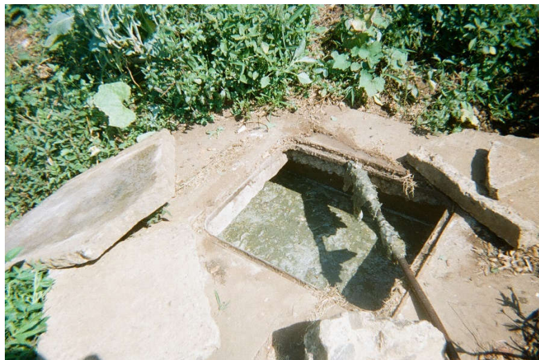
Figure 19 Picture taken by sewer worker as part of photo-elicitation exercise showing materials found in blockages
