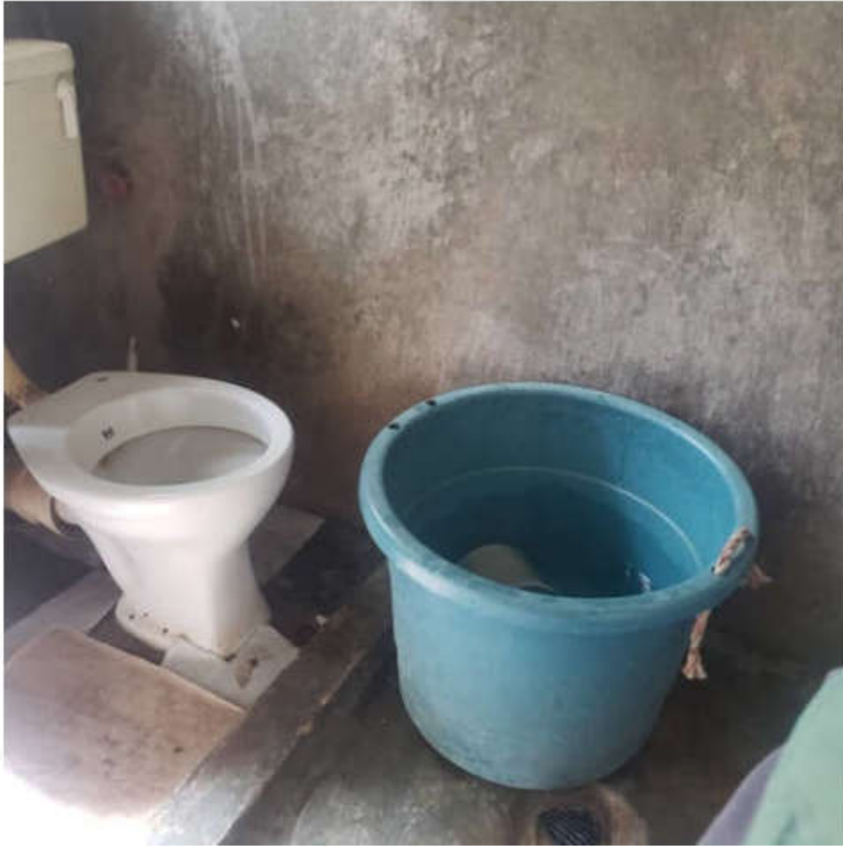
Water storage tub next to non-functional flush toilet in Lilongwe, Malawi. Photo: Ralph Ndalama, 2021
