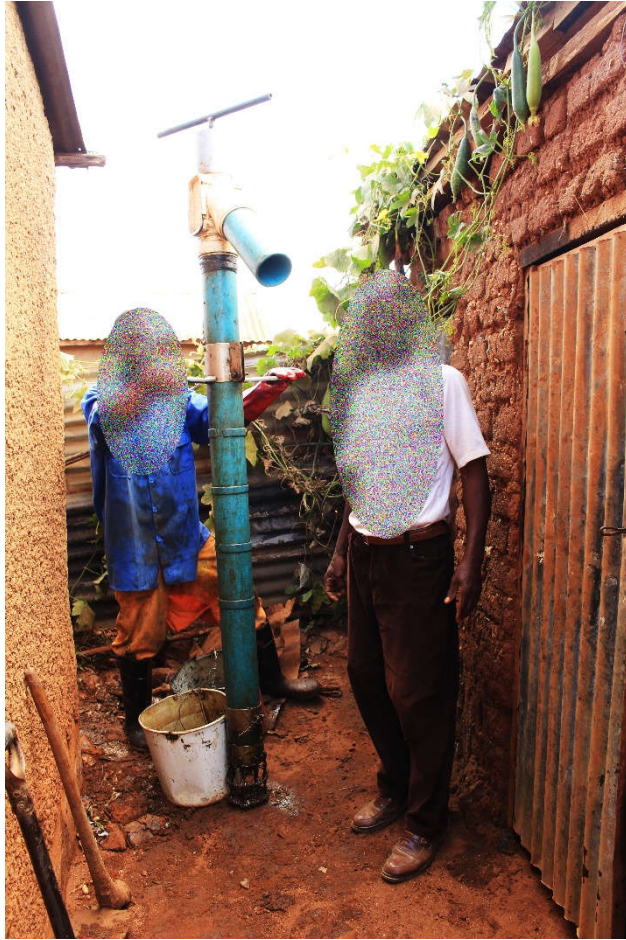
Figure 16 Latrine emptiers with gulper pump next to latrine in a LIA. Image: Author's Own
