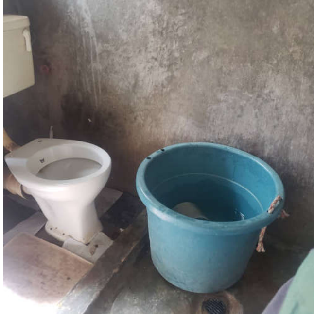
Figure 11 Water storage bucket next to non-functioning flush toilet in Area 18. Source: Ralph Ndalama, 2021. Used with permission.
