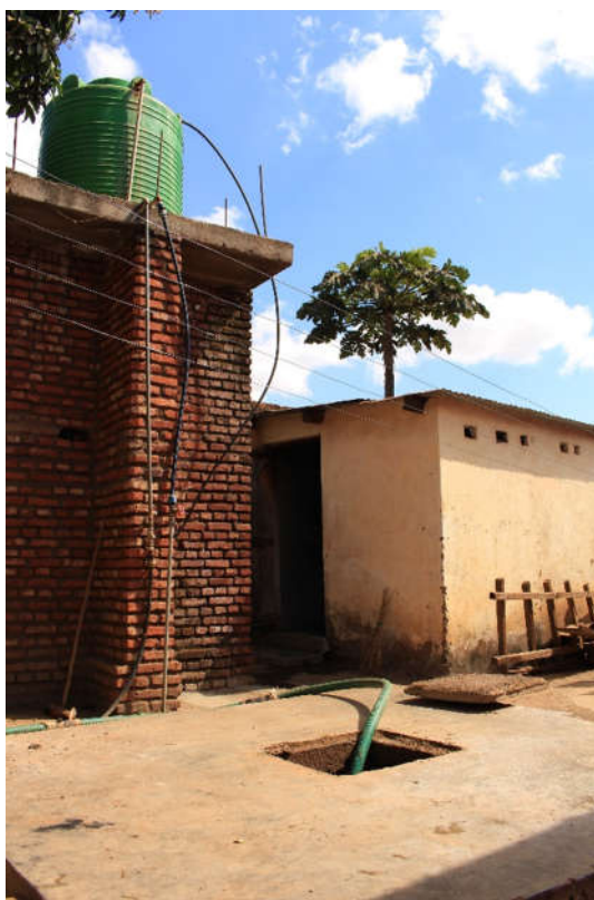
Figure 3. Coexisting infrastructures in the planned areas of Lilongwe. House with water tank to supplement network supply (left), backyard latrine and bathroom (right) and septic tank (front).
