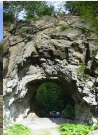
Fig. 9 Rail tunnel built – Tișiței Gorges
