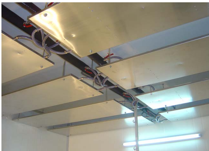
Photo 3.1c: Drop down type ceiling
