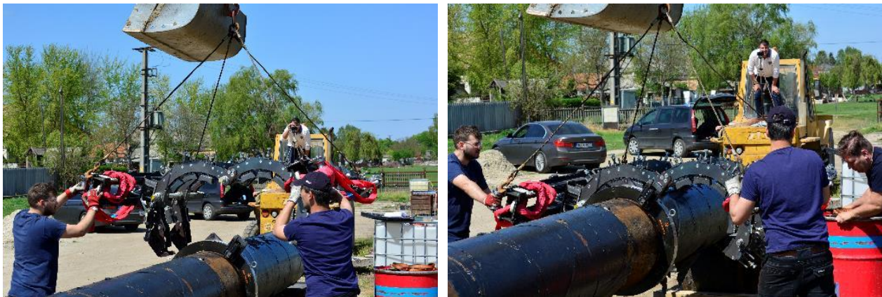
Figure 8. Installing the pipe positioning device
