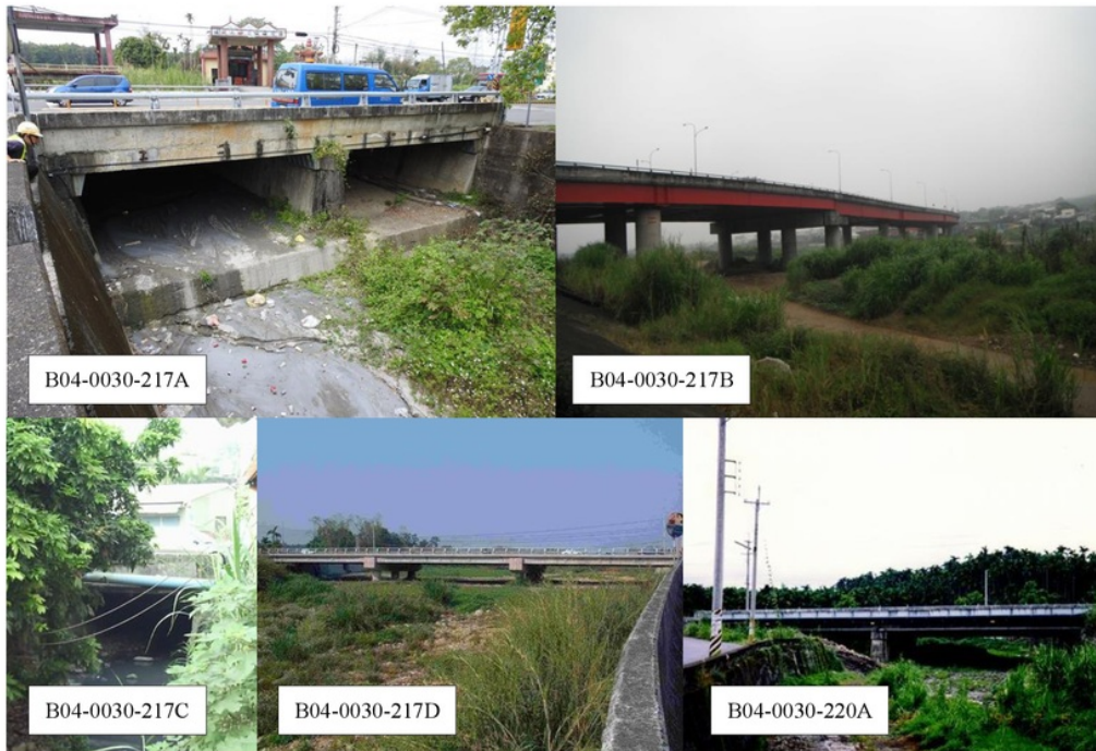
Fig. 4. Photographic documentation for each bridge obtained from TBMS database
