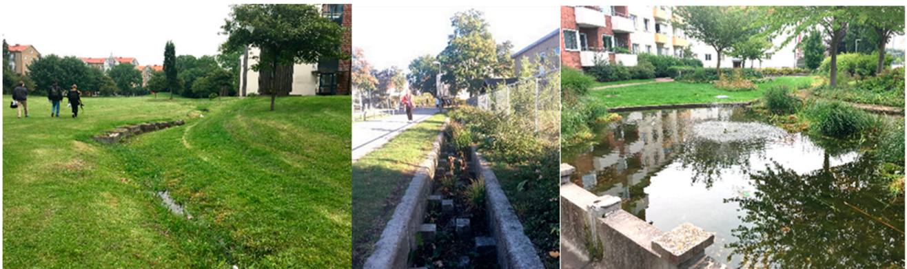
Figure 2. From left to right: Sunken lawn (Augustenborg remodelled park); sample of paved canal; sample of wet pond. Photographs by Misagh Mottaghi.
