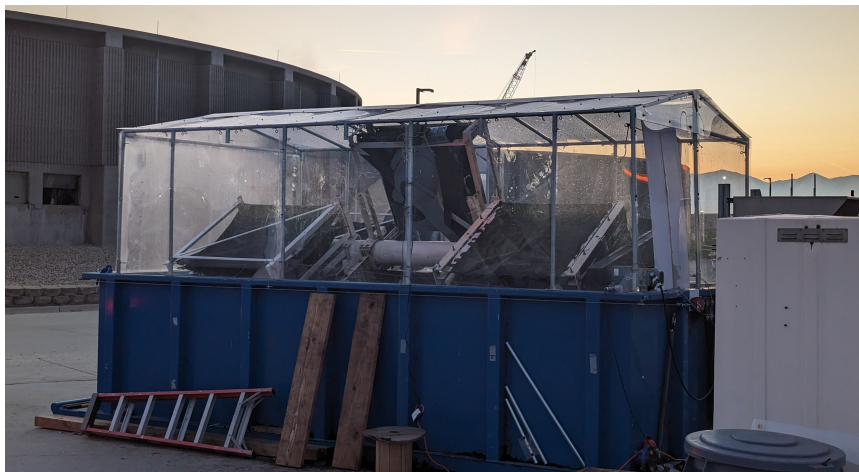
Figure 1.1: A side view of the pilot scale RABR operating at the Central Valley Water Reclamation Facility (CVWRF). The algae biofilm is grown on a square substratum sheet and rotated into a 4,500 L tank containing anaerobic digester effluent. A plastic polycarbonate cover has been mounted to reduce heat loss in the winter months.
