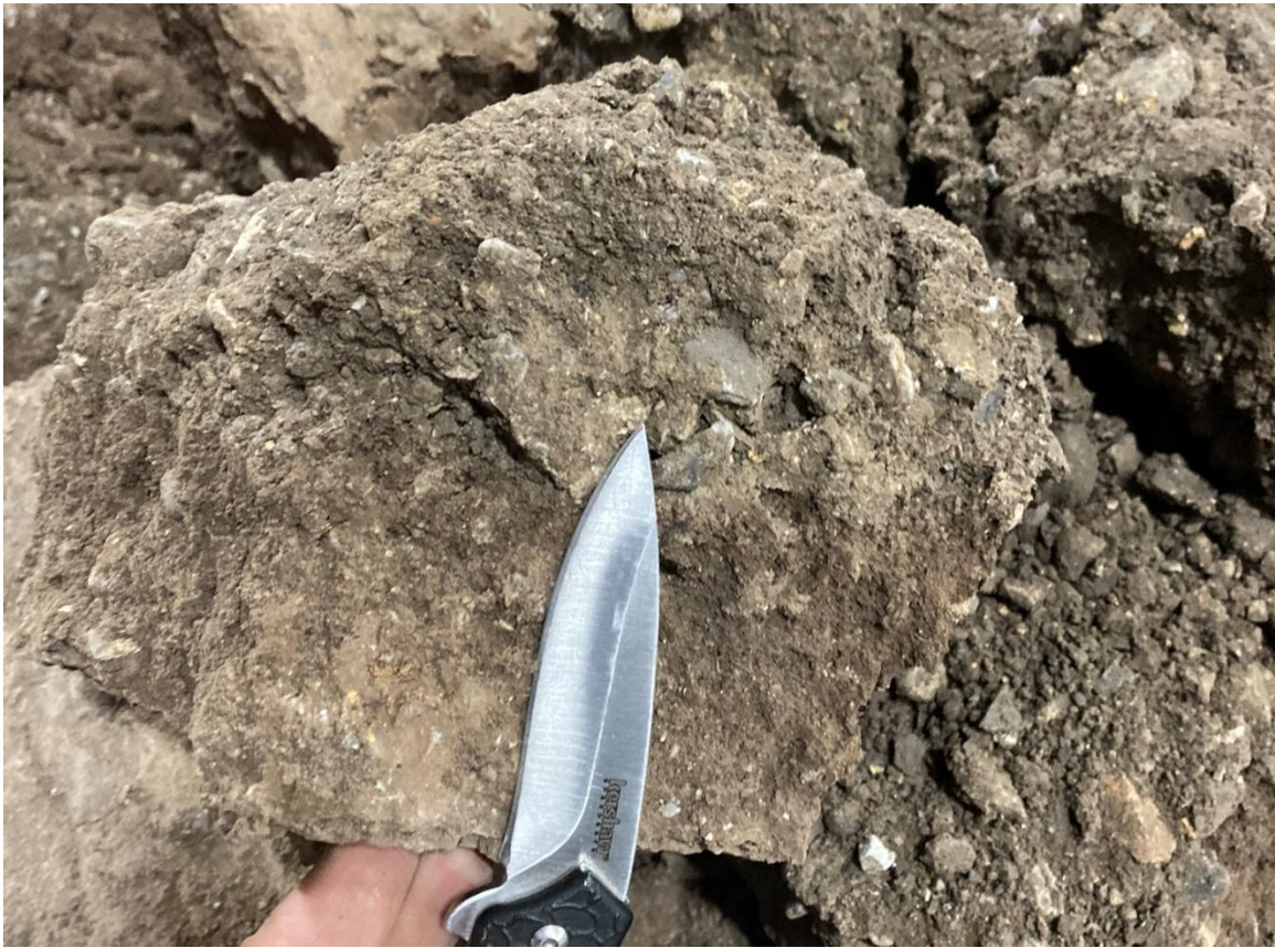
Fig. 26. Photo of topsoil and embankment fill bonding.
