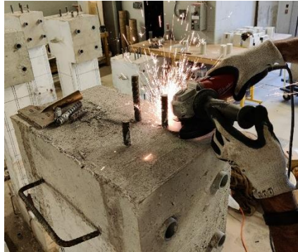
Figure 6-19. Removing extruded bars from the top of the columns.
