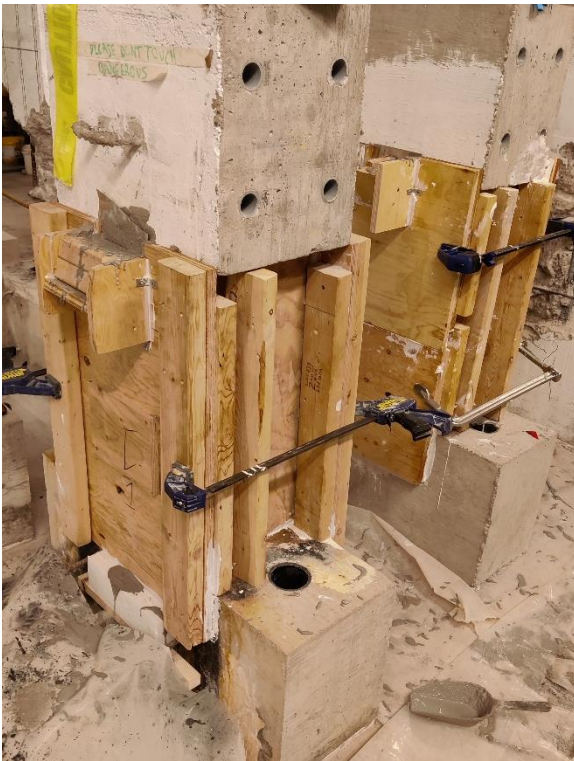
Figure 6-25. Sample of formwork used during the repair/strengthening process
