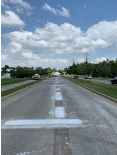
Partial Depth Concrete Joint Repair
