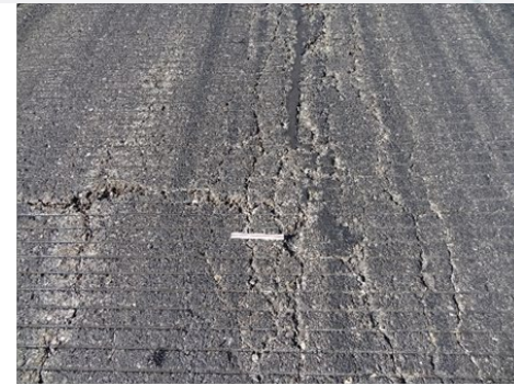
Alligator Cracking
