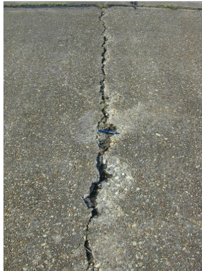
LTD Cracking
