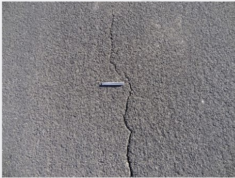
L&T Cracking
