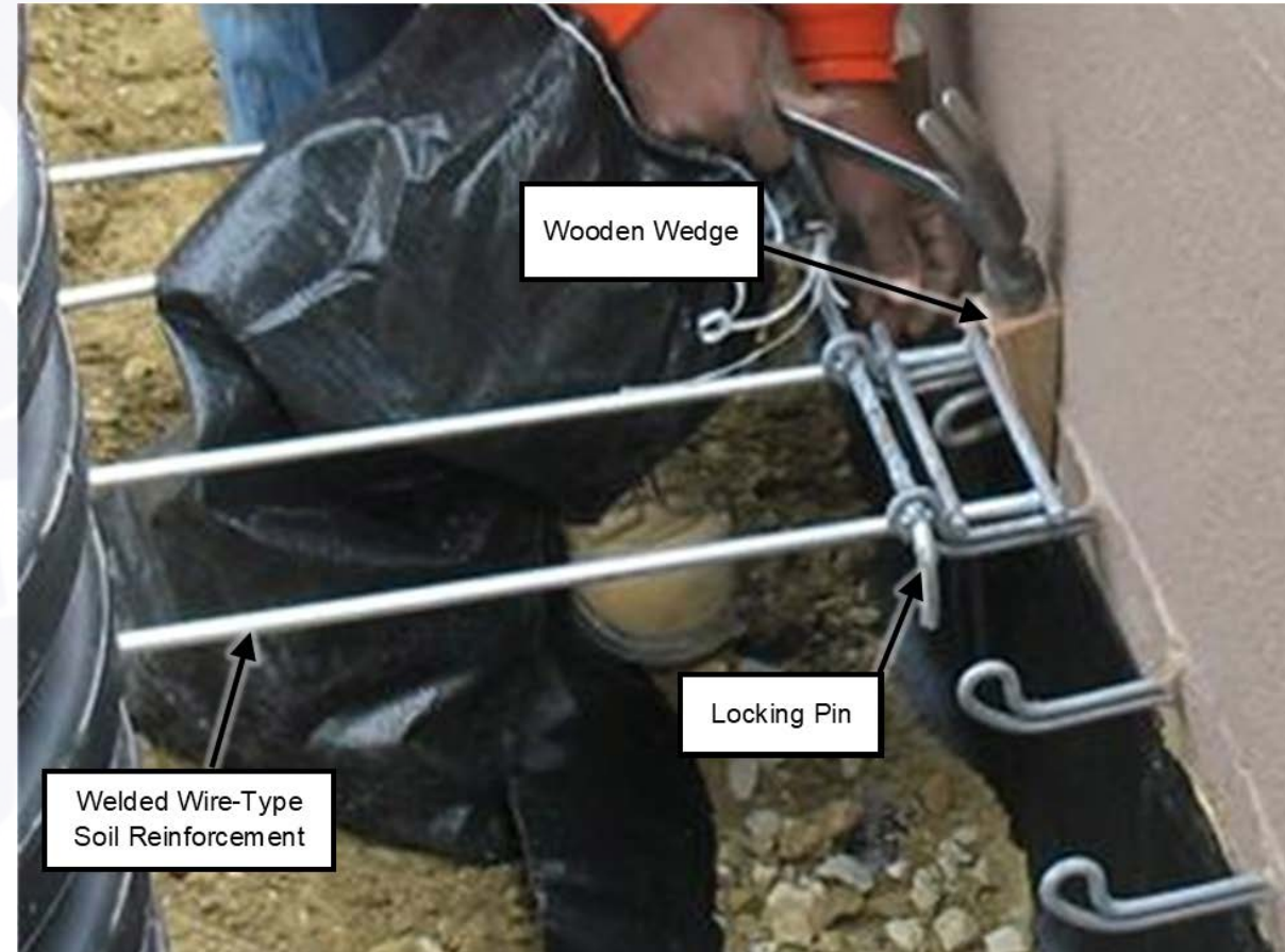
Example connection for welded wire reinforcement
