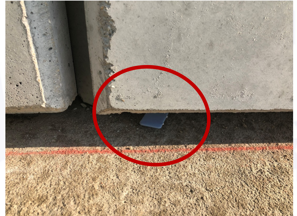
Typical MSE wall vendor supplied shims
