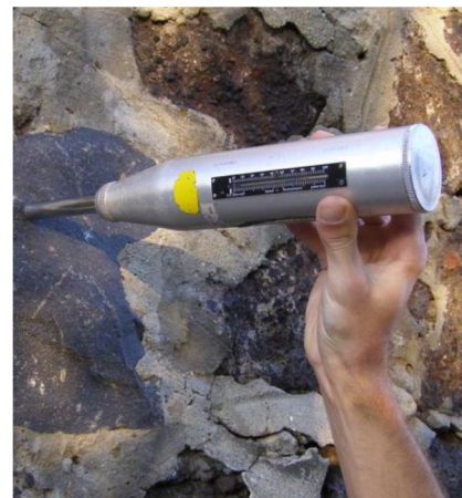
Fig. 1: Schmidt hammer strength tests.
