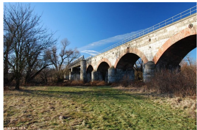
Fig. 5: View of the Marchegg Viaduct from the Slovak side.
