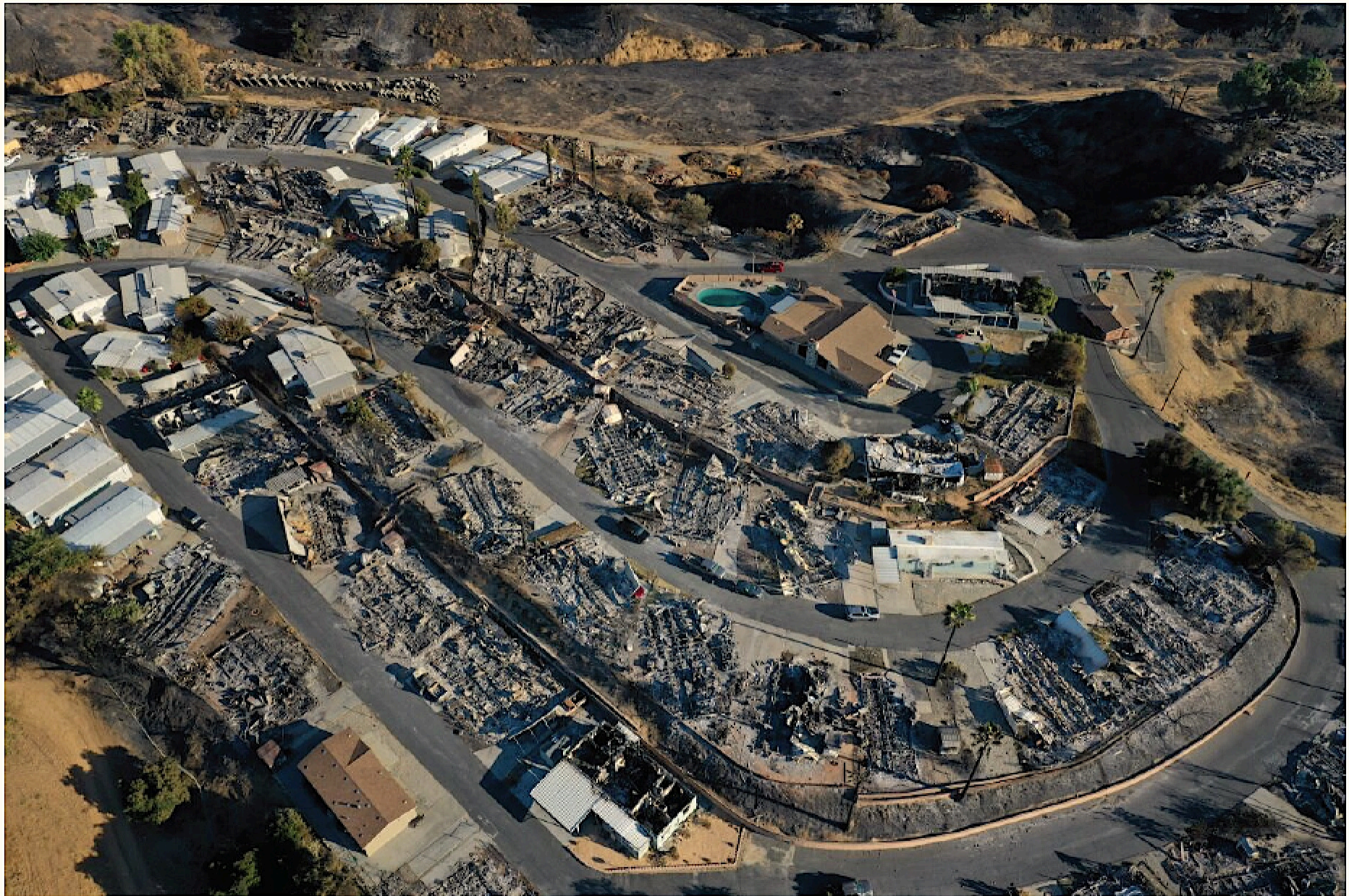
Aerial view of the Calimesa Mobile Home Park that was severely damaged in the Sandalwood fire. (Carolyn Cole/Los Angeles Times)
