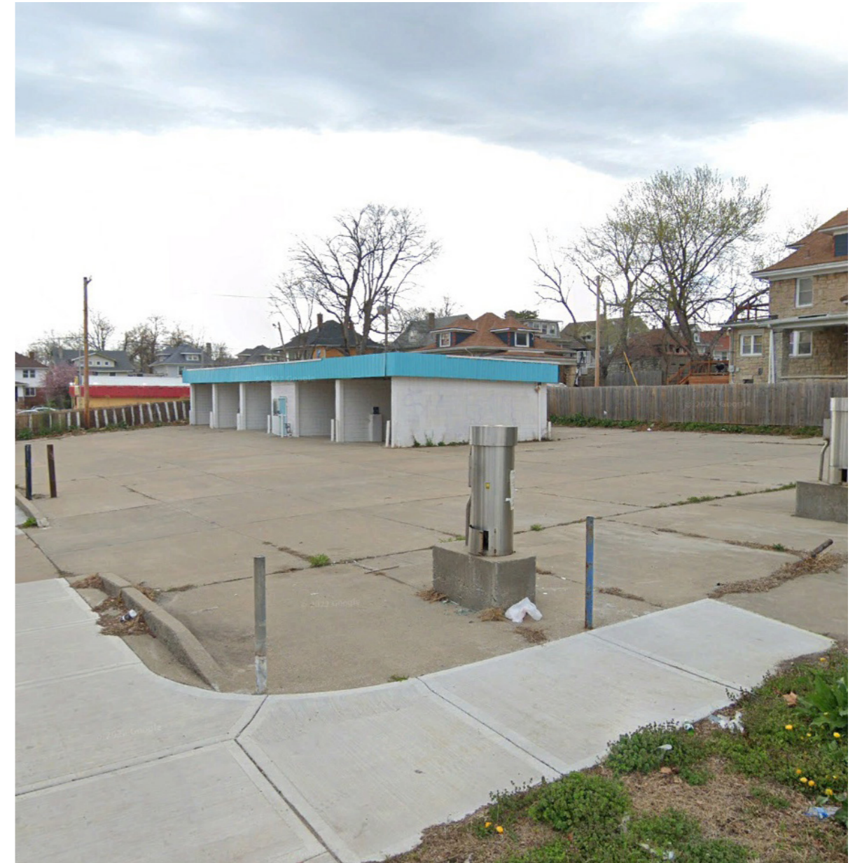
Figure 3.7: Post commercial vacant lot with paving and structure from its previous use.
