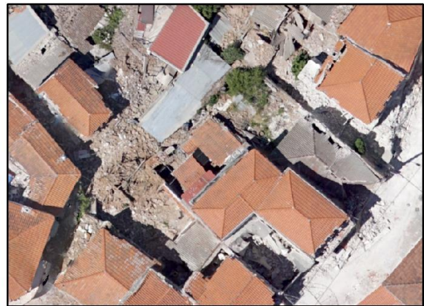
Figure 6. Part of the 13 th June 2017 orthophoto map at a scale of 1:500 with damages of grade 4 e.g. heavy structural failure of roofs and floors.
