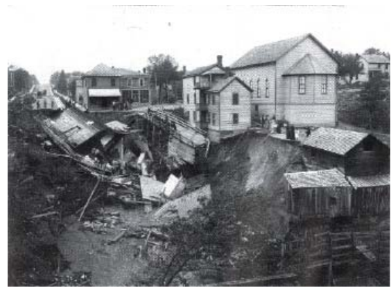
Landslide on Myrtle Street
