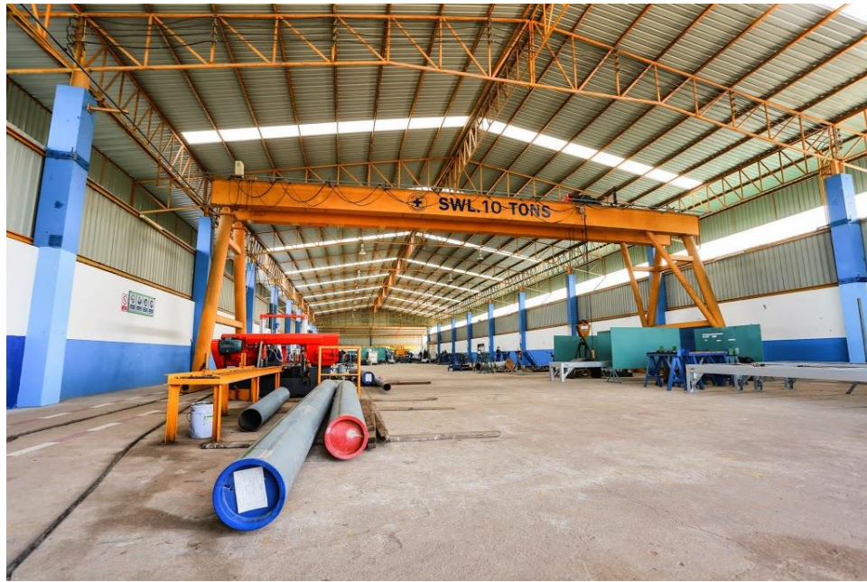
Figure 13 The inside workshop building.
