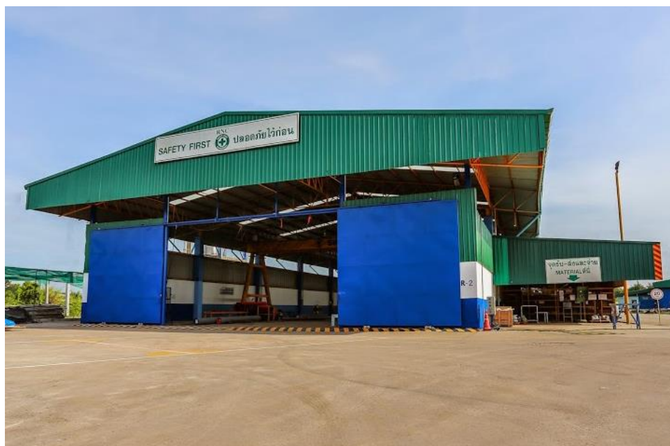
Figure 12 The workshop building.
