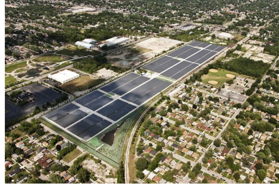
Figure 6.2. Exelon City Solar, Chicago Illinois (Source: Turner Constructions)
