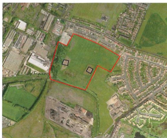
Figure 5.1. A typical brownfield site at Cromdale Gove with amenity grassland on shallow soil (10-30 cm depth) overlying a former landfill site that received domestic, industrial and chemical waste (including colliery spoil, ash and rubble) in the 1960s and 1970s surrounded by residential buildings and light industry (French et al., 2006)
