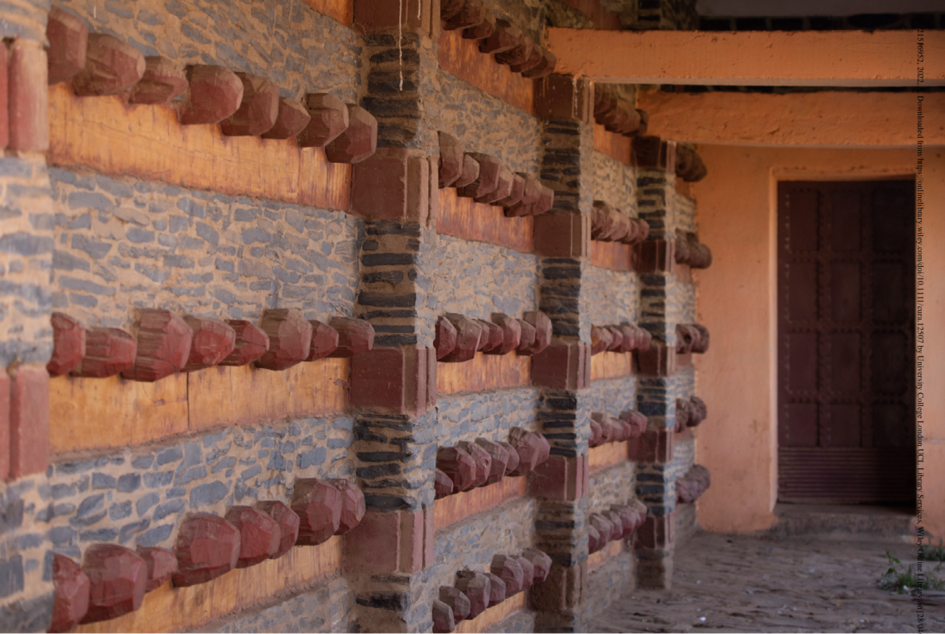
Figure 16. The Deghe Selam alternating slate and wood layers in monkey head style, designed by Odoardo Cavagnari, 1917. Biniam Teame's personal archive, 2022. [Color figure can be viewed at wileyonlinelibrary.com ]
