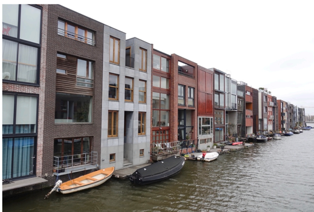
Fig. 10. Borneo Sporenburg, Amsterdam, in this development, the code allowed considerable architectural freedom within a unifying framework. The code defined by West 8 controlled height to the eaves, number of stories, height of the first storey (4.5 m) the roof (it should be flat), and the pallet of materials (Image: Matthew Carmona).
