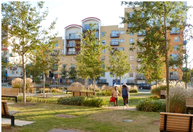
Fig. 33. High quality placemaking at Greenwich Millennium Village, tested in the first round of pilots. The design code in this case provided the wireframe to structure successive phases of the development over 25 years (image: Matthew Carmona).
