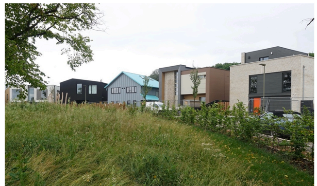
Fig. 25. Plot passports are being used at Graven Hill Village, Buckinghamshire, to guide the design of self-built plots. These offer a good degree of architectural flexibility within a common urbanistic wireframe provided by the village design code (image: Matthew Carmona).
