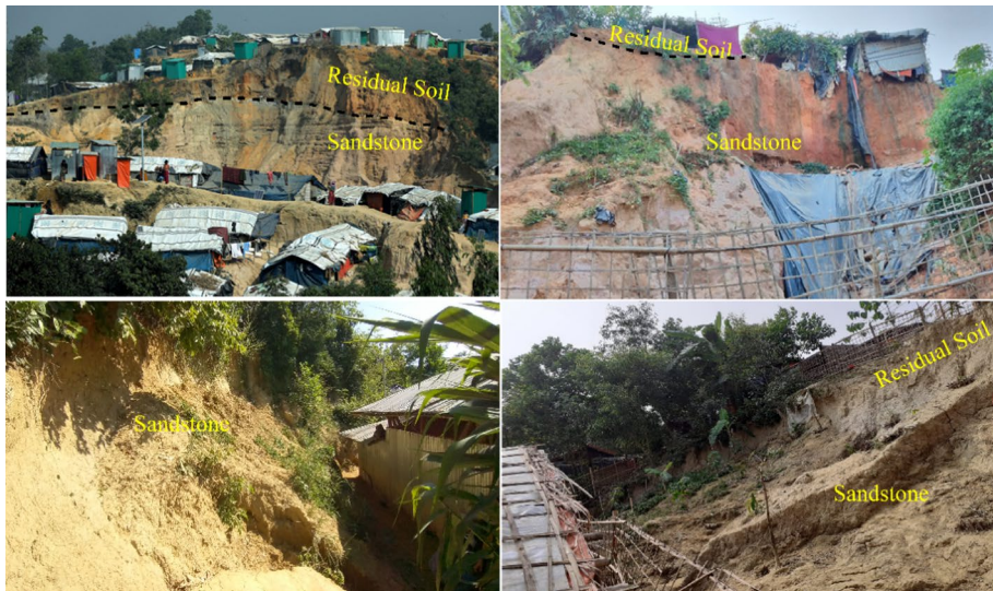
Fig. 2 Landslides in the Kutupalong Rohingya camp
