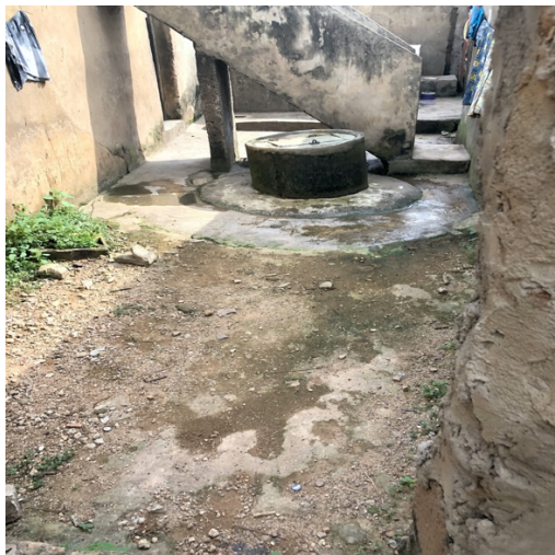
Figure 12: Image portraying the staircase that leads to P06's bathroom outside
