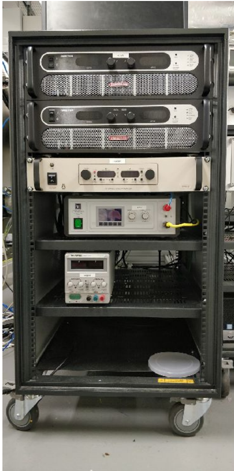
Figure 5.14: The power supply rack showing from top to bottom: two anode power supplies, the keeper power supply, heater power supply and magnet power supply. Please see text body for model numbers and specifications.
