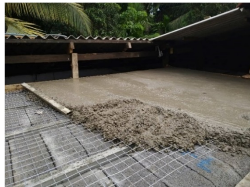
f) casting of screed over reinforced slab system
