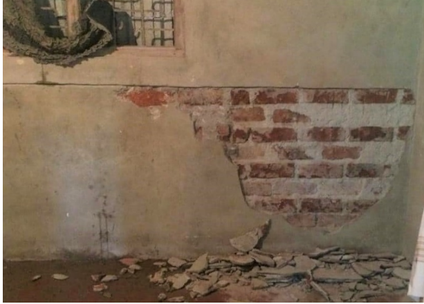
a) removal of existing plaster
