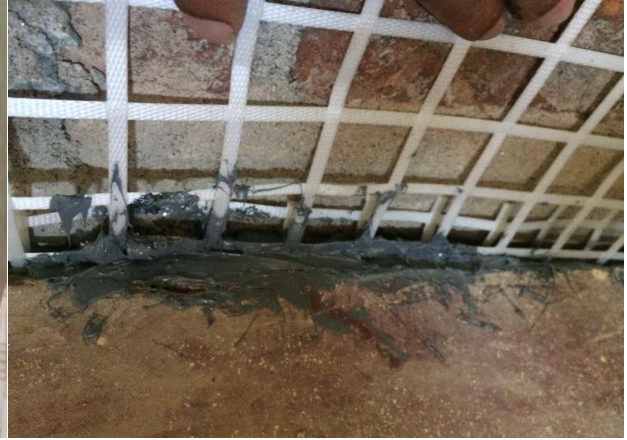
b) epoxy the geogrid in place
