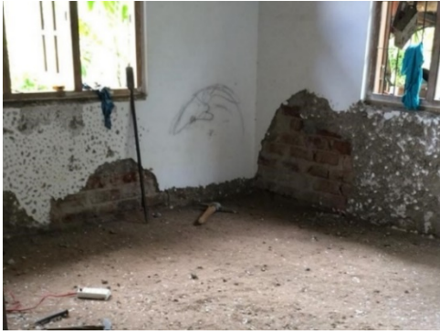
a) existing wall and floor plastering removed
