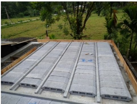
e) installation of inverted-T beams and infill
