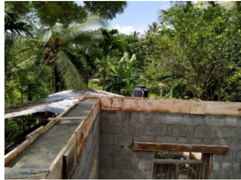
d) walls capped with reinforced ring beam
