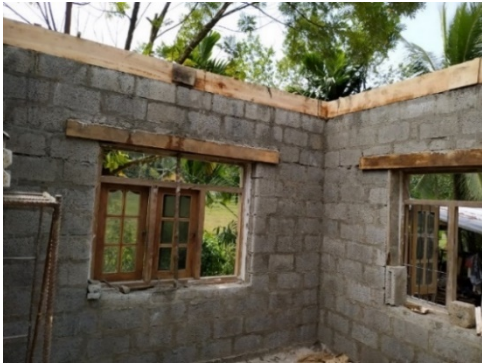
c) ground floor walls with lintel beams added
