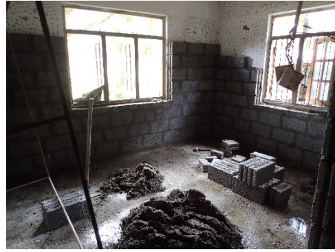
b) construction of interior wall
