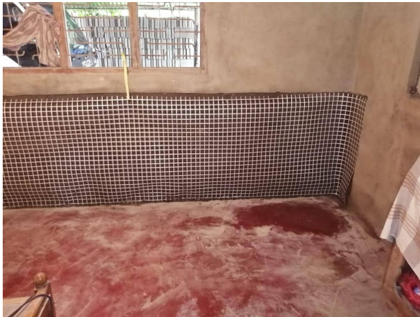
c) application of scratch coat and geogrid
