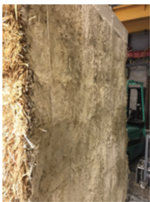
Figure 4 Initial key coat of lime plaster
