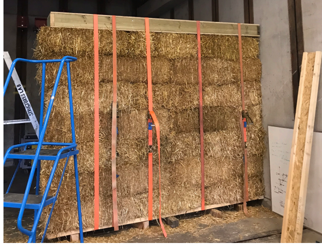
Figure 3 Three-bale straw bale wall during pre-compression
