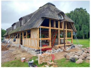
Figure 9.6 Almarksvej 2, Horne. Private client. Total renewal of an old farmhouse, no stone untouched. The thatched roof is only kept as a temporary cover during the reconstruction. Photo & Project work 2022/PJA
