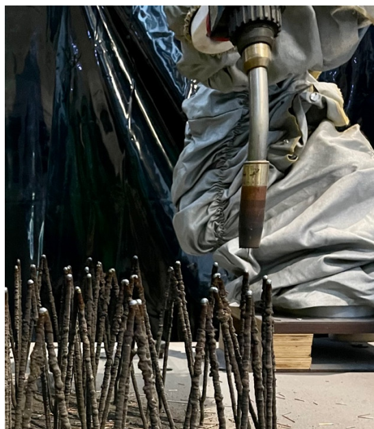
Figure 6. Printing process of a WAAM lattice structure.
