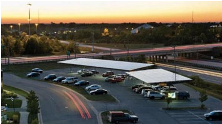
Figure 12. Solar Canopy in Parking Lot (Michigan)
