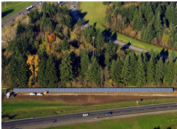
Figure 9. Solar Array at Highway ROW (Oregon)
