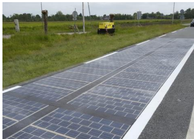
Figure 13. Solar Pavement - Wattway by Colas (France)
