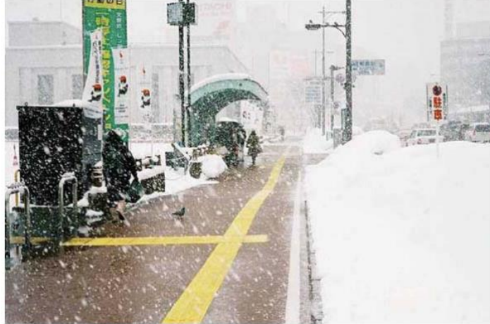
Figure 14. Sidewalk heating in Aomori City, Japan – condition on the snow-melting section in December 2002
