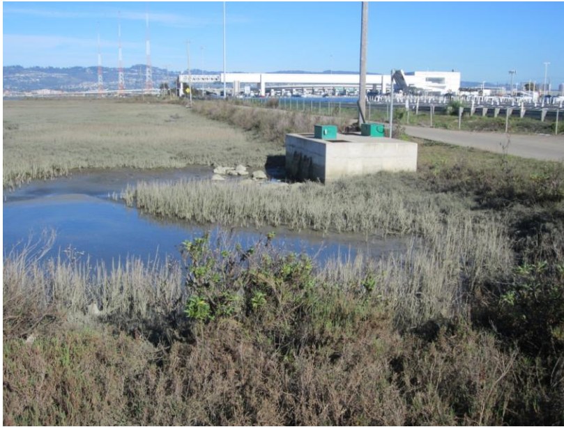
Figure 5-12: A site photo (looking east) of the dirt access road adjacent to I-80. One of many drainage structures owned and operated by Caltrans, can be seen adjacent to the road
