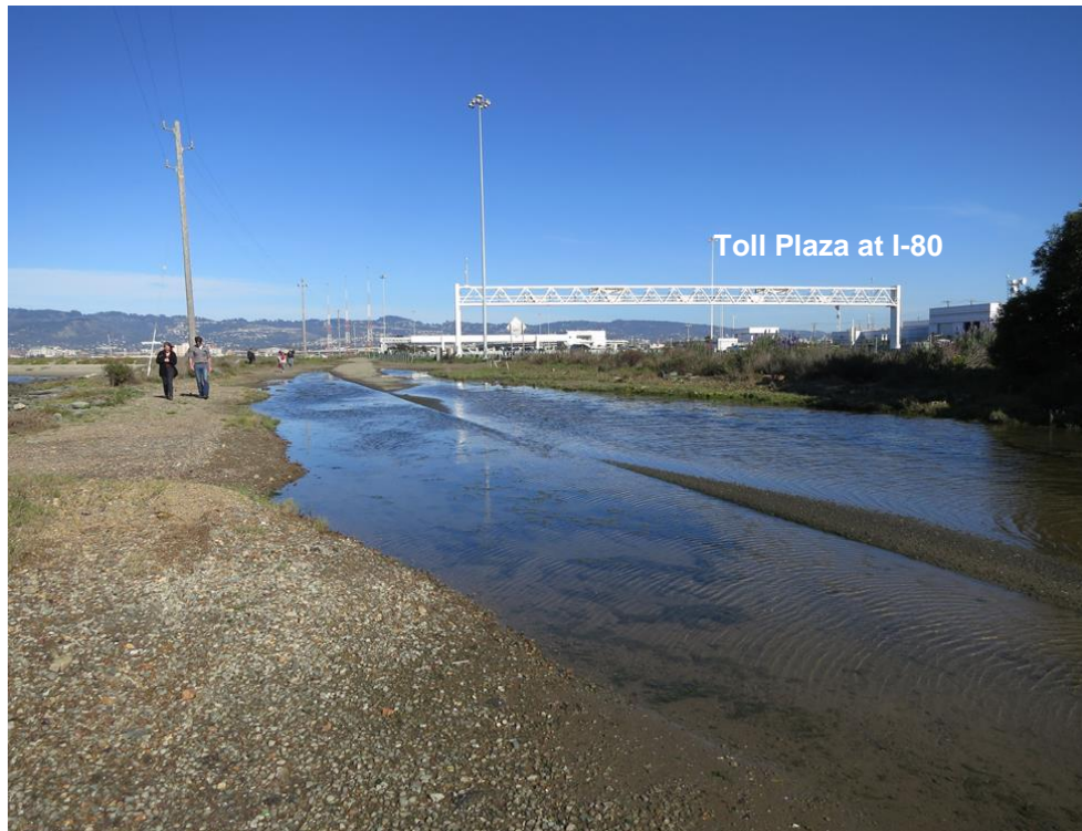
Figure 5-9: Cross-shore profile of the inundated access road adjacent to I-80, immediately west of the toll plaza under MHHW + 36 inches SLR conditions
