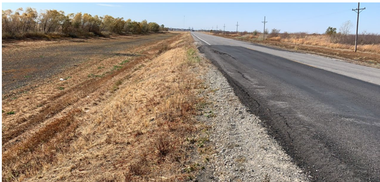
Figure 3-1: Example of an embankment inventoried in the MoDOT GAM program.
