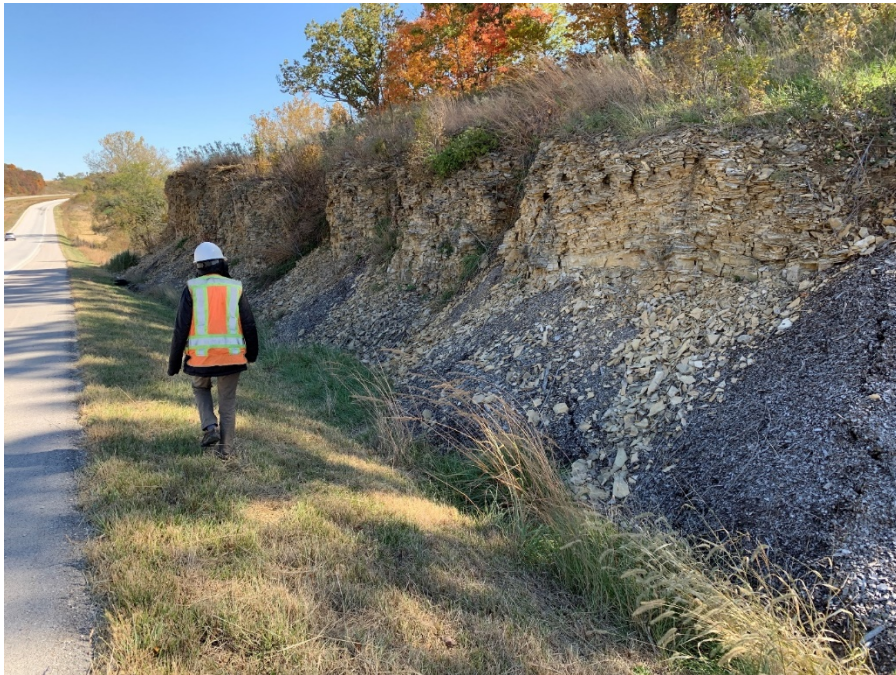
Figure 3-4: Example of a rock slope that was not inventoried in the GAM application because the slope height was less than the ditch width.
