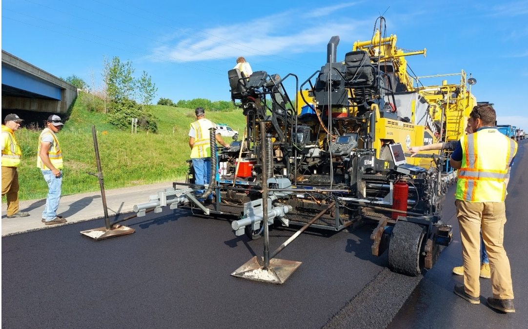
Figure 28. Demo No. 2 -ARTS data collection during paving.
