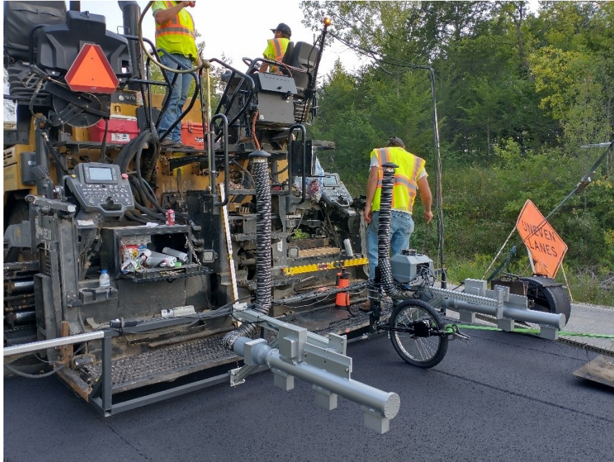
Figure 9. Demo No. 1 - ARTS sensor set up and operation.
