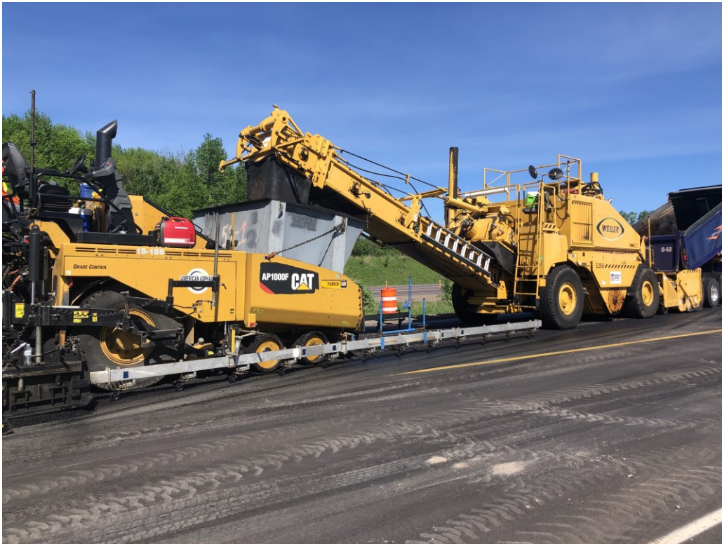
Figure 25. Demo No. 2 – Truck, MTV, and Paver Operations.
