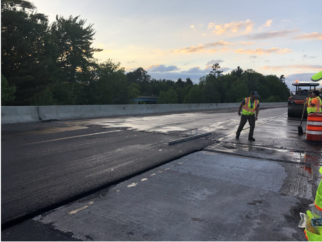
Figure 32. Demo No. 2 – Bridge Deck Tied-in.
