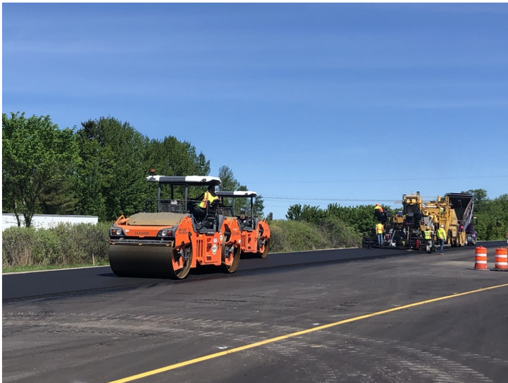
Figure 27. Demo No. 2 – Roller Compaction.
